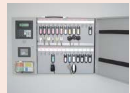
RFID entry control system
